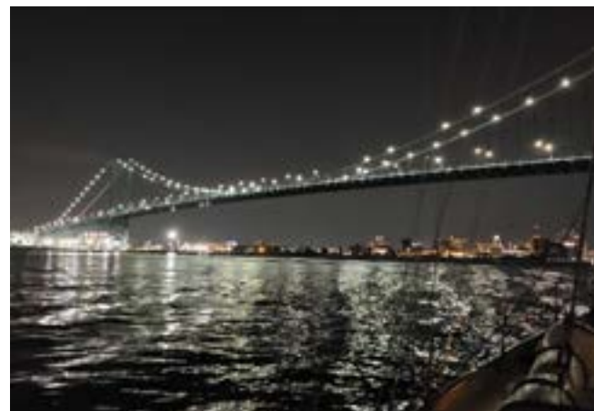
July 4th going up the Detroit River. Come on, come on BABY! Why Ted? In 2021 we rocked to a Detroit/Michigan playlist for our 7 kt sail upstream past Cobo Hall. Mr. Nugent rocked!
