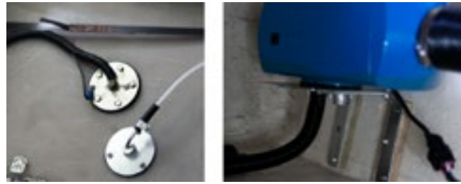
left: Tapping into the diesel tank . right: installation process.
