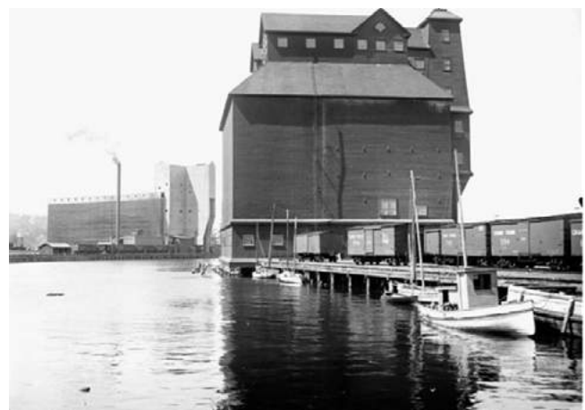
Original Midland City Grain Elevator - Topley Studio / Library and Archives Canada / PA-008550
